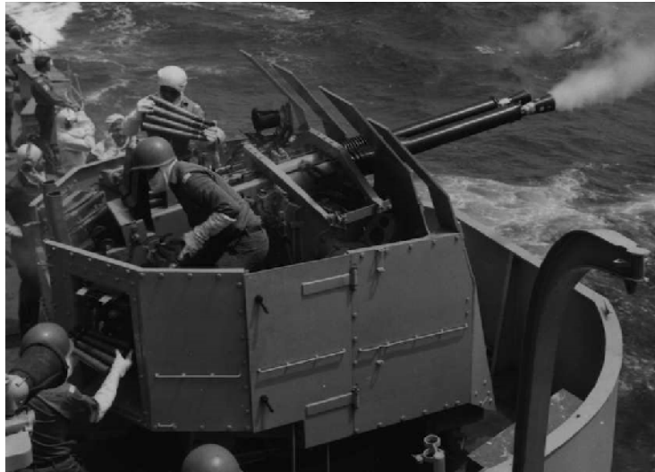
The British-built Bay Class frigates were fitted with the twin 40mm Mk V powered mounting. This one is on the Tribal Class destroyer HMAS Arunta . Note that the ammunition supply still requires crew to follow the mount and pass four rounds at a time up to the loaders. [navy.gov.au]
