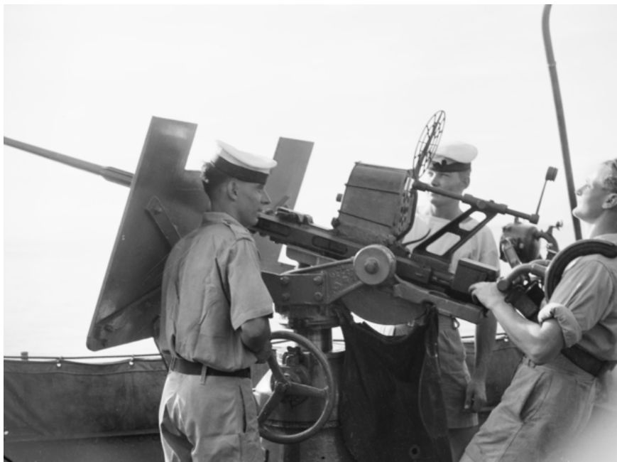
The 20mm Oerlikon with the hydraulically-adjustable Marks 1, 1A and II (US Marks 2 & 4) mounts that required the extra man and a certain amount of teamwork. Note the wheel on the left-hand side to raise the gun and the sailor manning it is co-ordinating with the gunner to achieve the correct elevation. The third seaman is ready to change the 60-round magazine.– in this case on an RAN Fairmile off Bougainville, 1945. [Australian War Memorial 095088]
