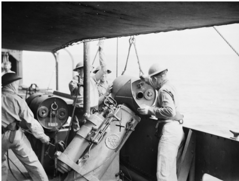
Depth charger being loaded from its storage rack on to a Mark III depth charge thrower on the corvette HMAS Geelong . [Australian War Memorial 075719]
