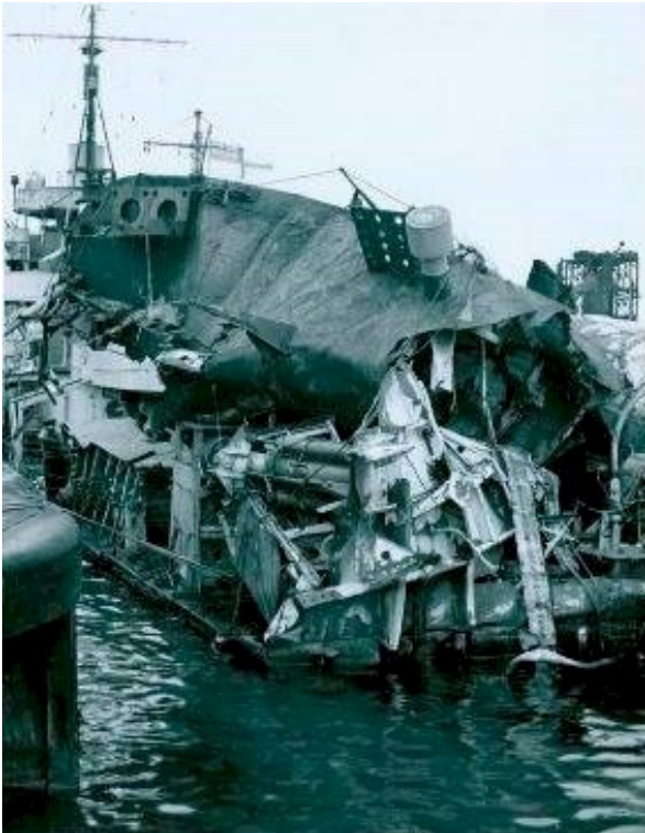
Damage to the port side of HMCS Chebogue . [forposterityssake.ca]
