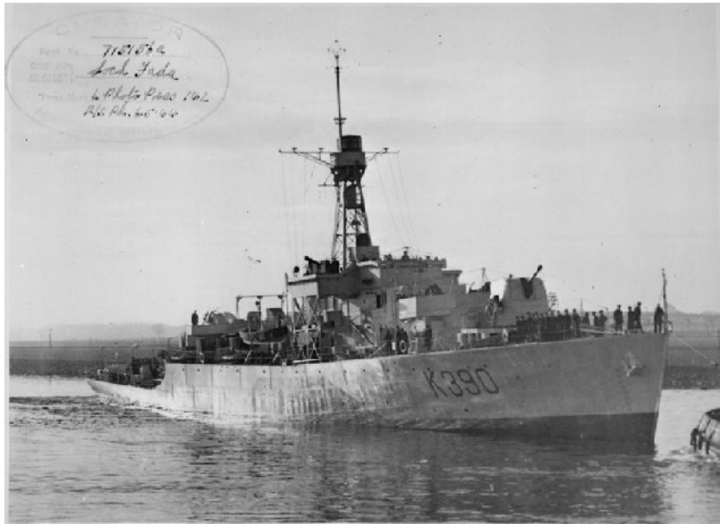
HMS Loch Fada , the first one laid down and essentially the prototype for the construction method, shortly after commissioning. Note she is fitted with the Type 272P radar in a teak and perspex lantern at the top of the lattice mast with the HF/DF antenna well above it. [en.wikipedia.org]
